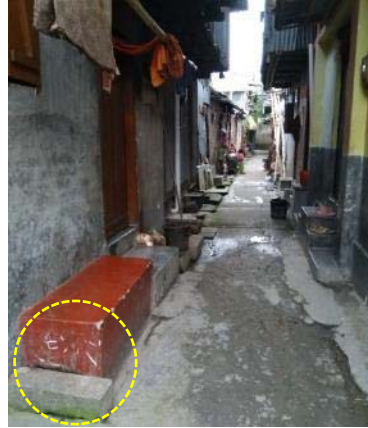
single pit connected to covered (operable) drain
